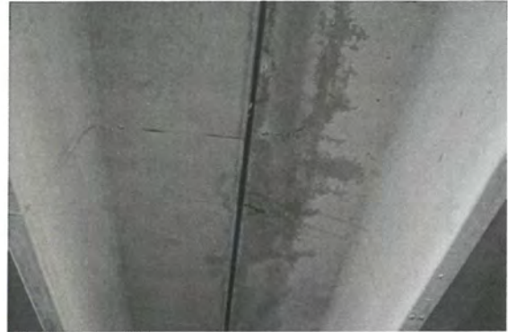
Photo 8: Typical water staining and active leaking
