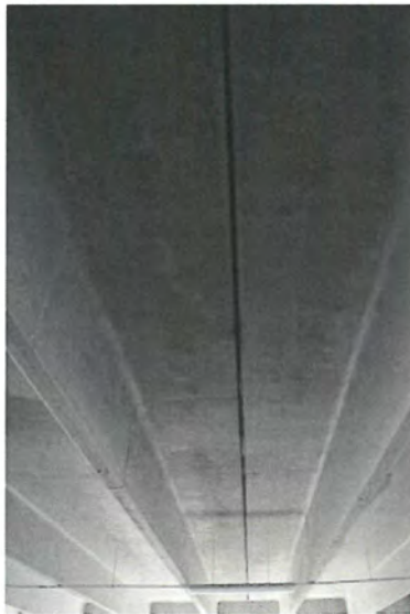
Photo 9: Typical water staining
