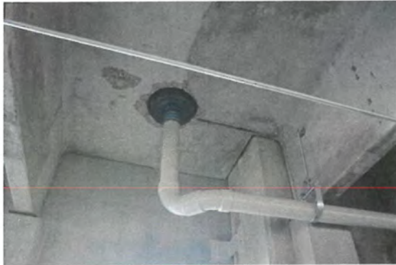
Photo 13: Minor spalling at utility penetration
