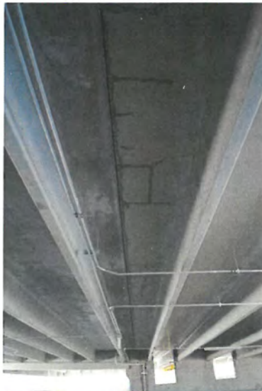
Photo 5: Typical water staining
