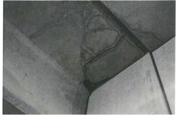
Photo 2: Cracked flange with exposed rebar
