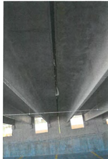
Photo 6: Membrane slipped through joint
