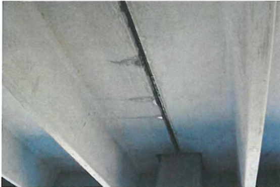
Photo 7: Typical water staining and active leaking
