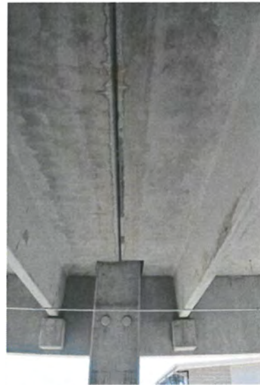
Photo 10: Typical water staining and active leaking
