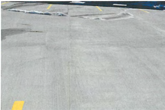
Photo 11: Cracks in wearing surface
